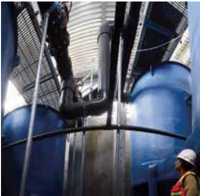
Ellie Key '01 inspects tertiary filters that remove phosphorus from secondary wastewater effluent.
